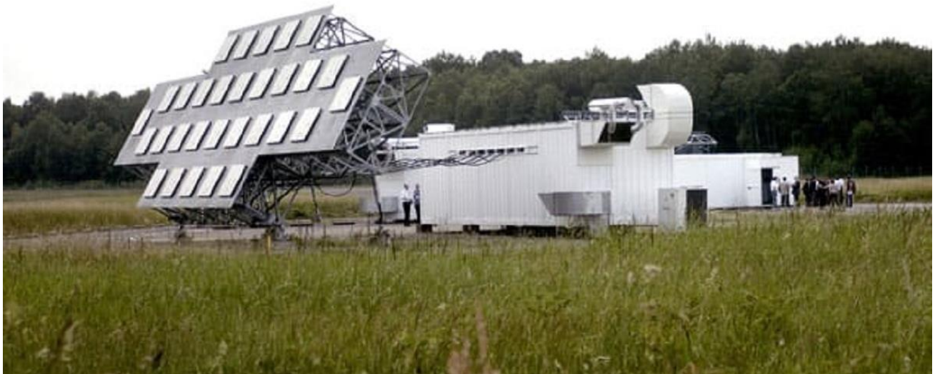
Figure 2 – The military radar at Graves, near Dijon, France.
