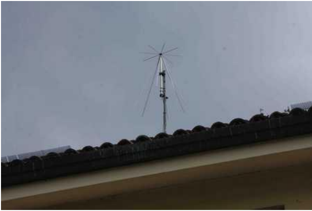
Figure 14 – “Discone” antenna.
